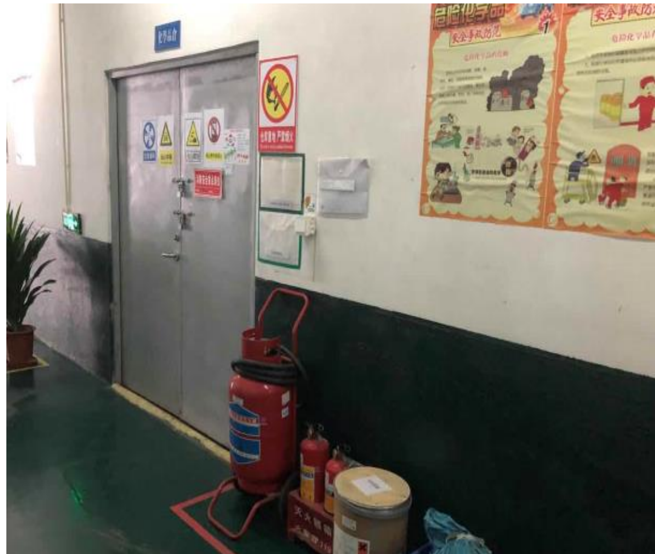
Fire-fighter equipment in chemical storage area
